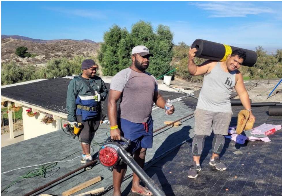
The Brothers working on the roof of the Main House here in Hemet, California.
